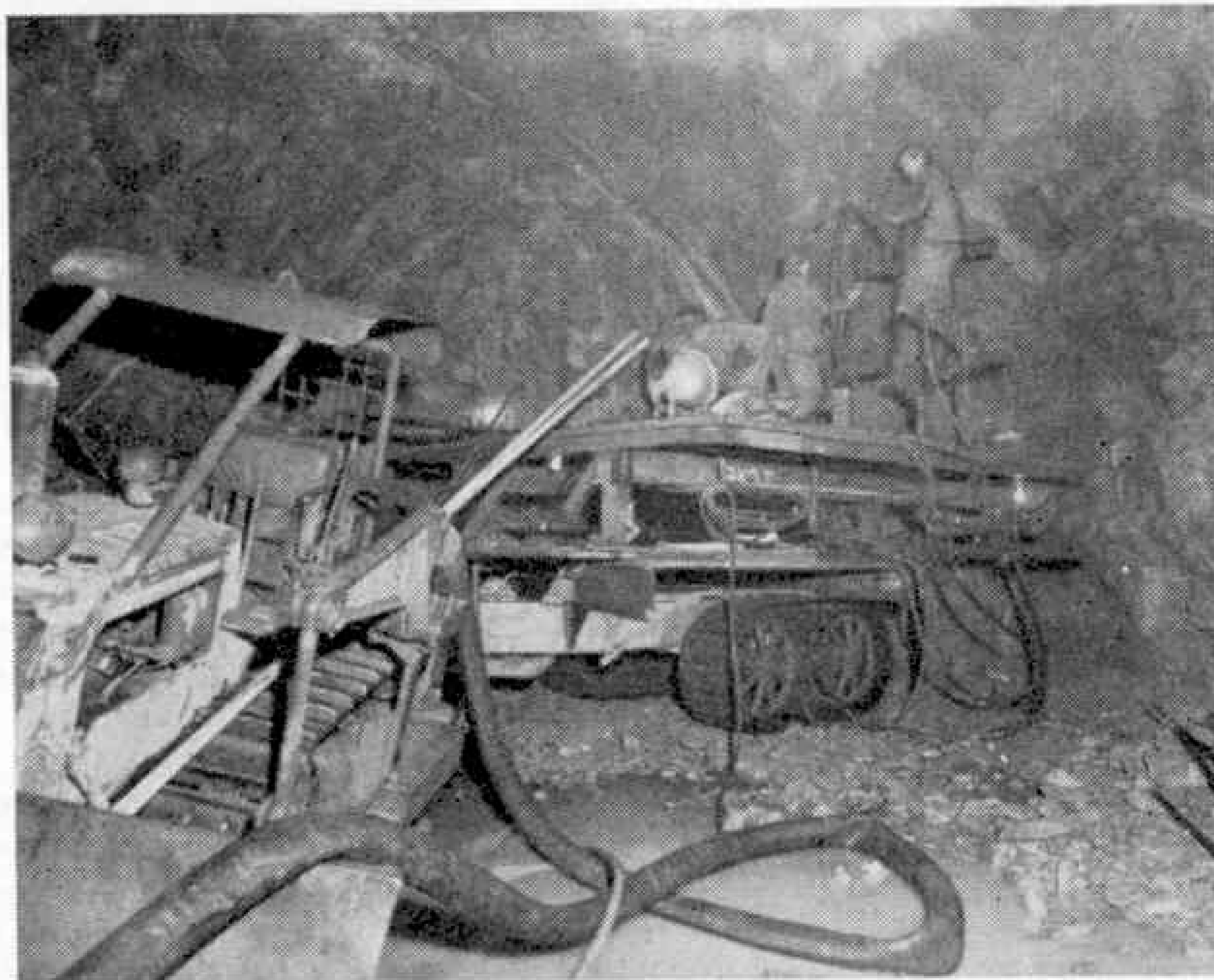
Setting up for drilling in one of the tunnels of the Kitimat project.
