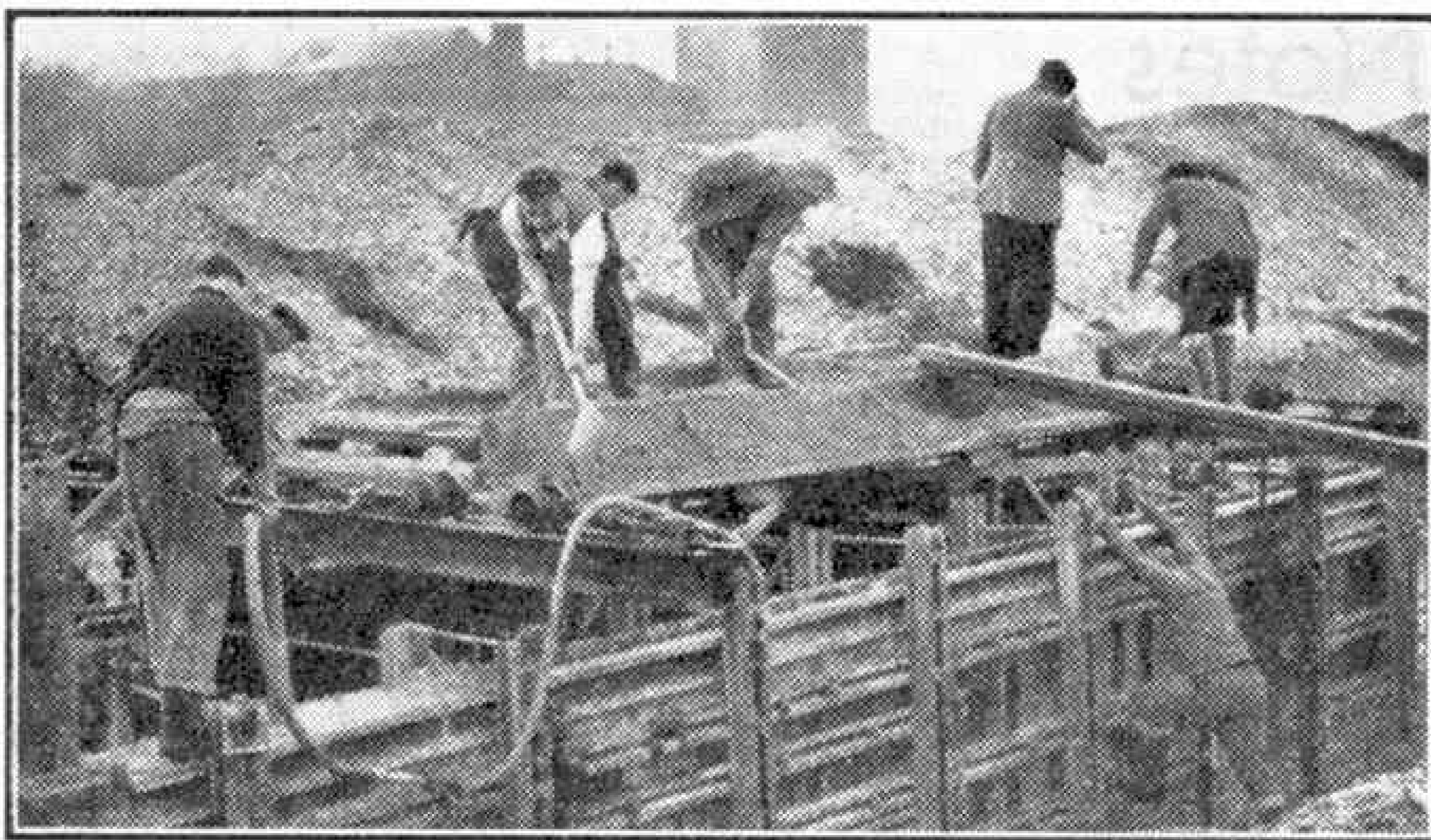
Fig. 8. Reinforced concrete storm water culvert under construction.
