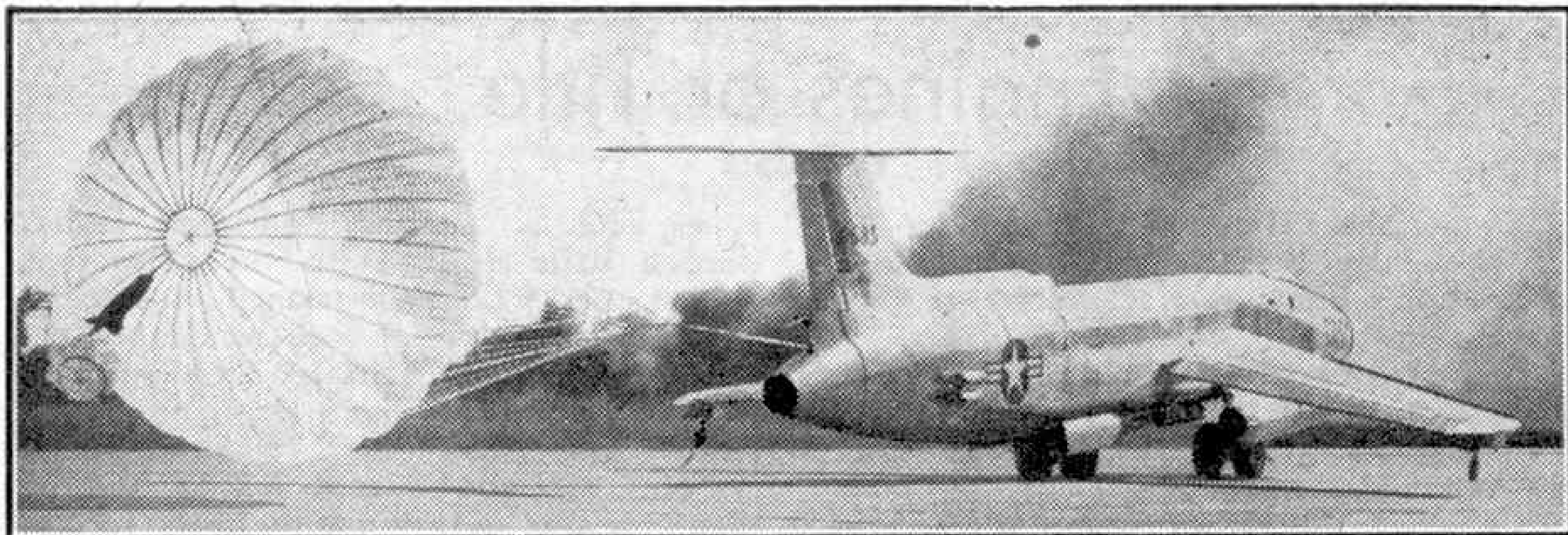
One of the first pictures showing use of the unique parachute braking technique on the new Martin XB-51 3-jet bomber. Photograph by courtesy of The Glenn L. Martin Co., U.S.A.
