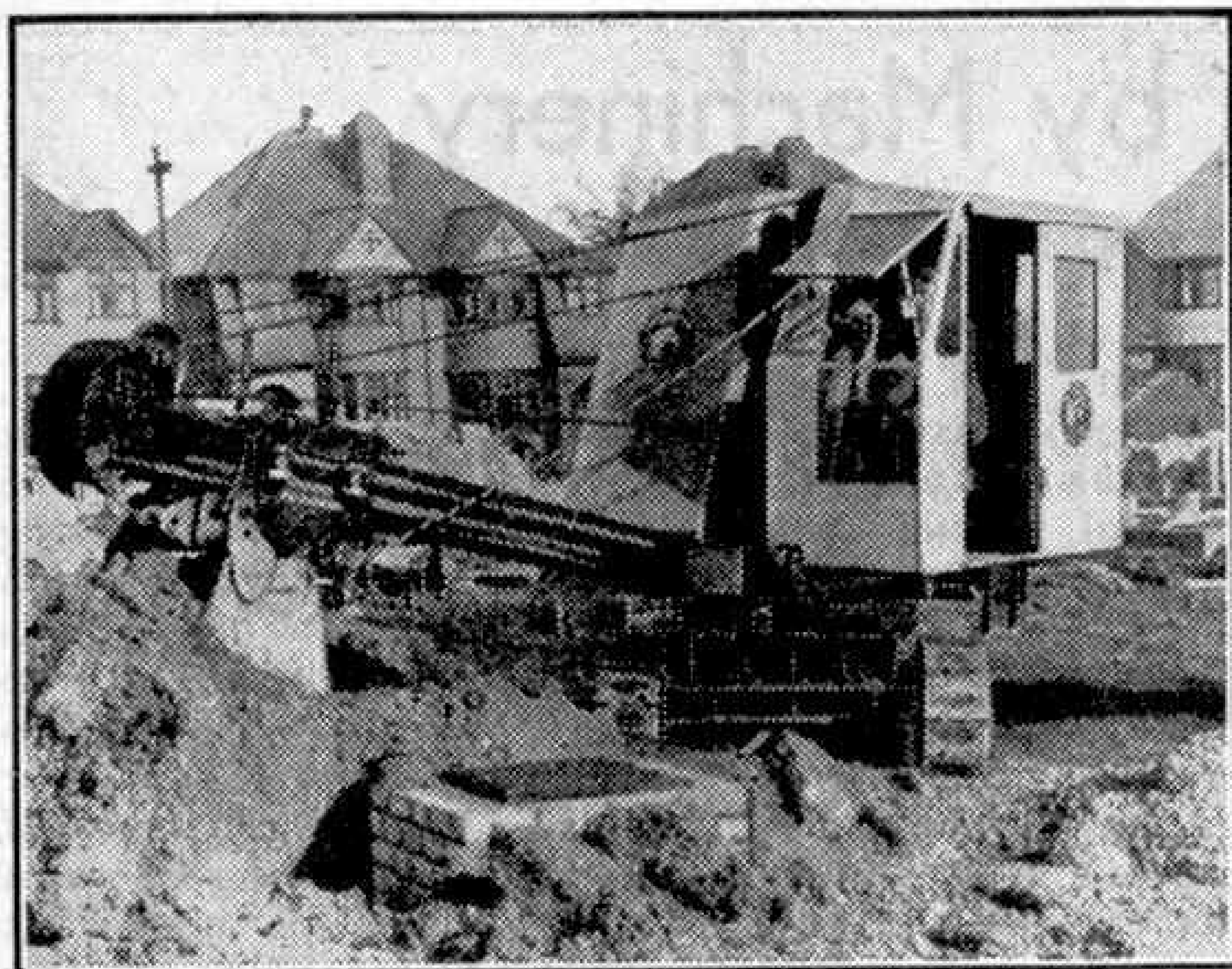
"Wolf" excavator, weighing 9½ tons, with a Skimmer attachment, levelling a road site on a housing estate.
