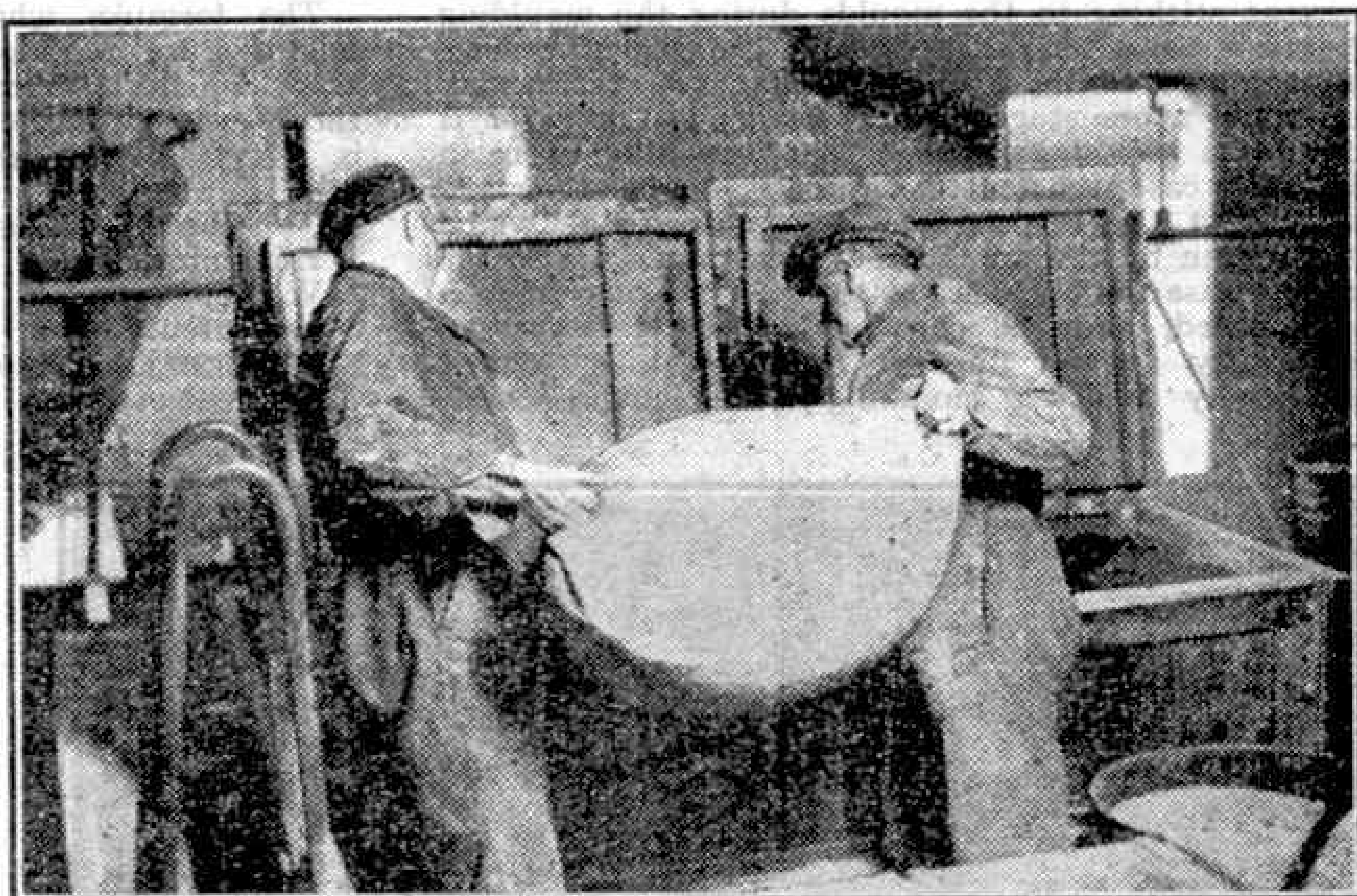
Filling the mixing machines prior to the dry mixing process.
