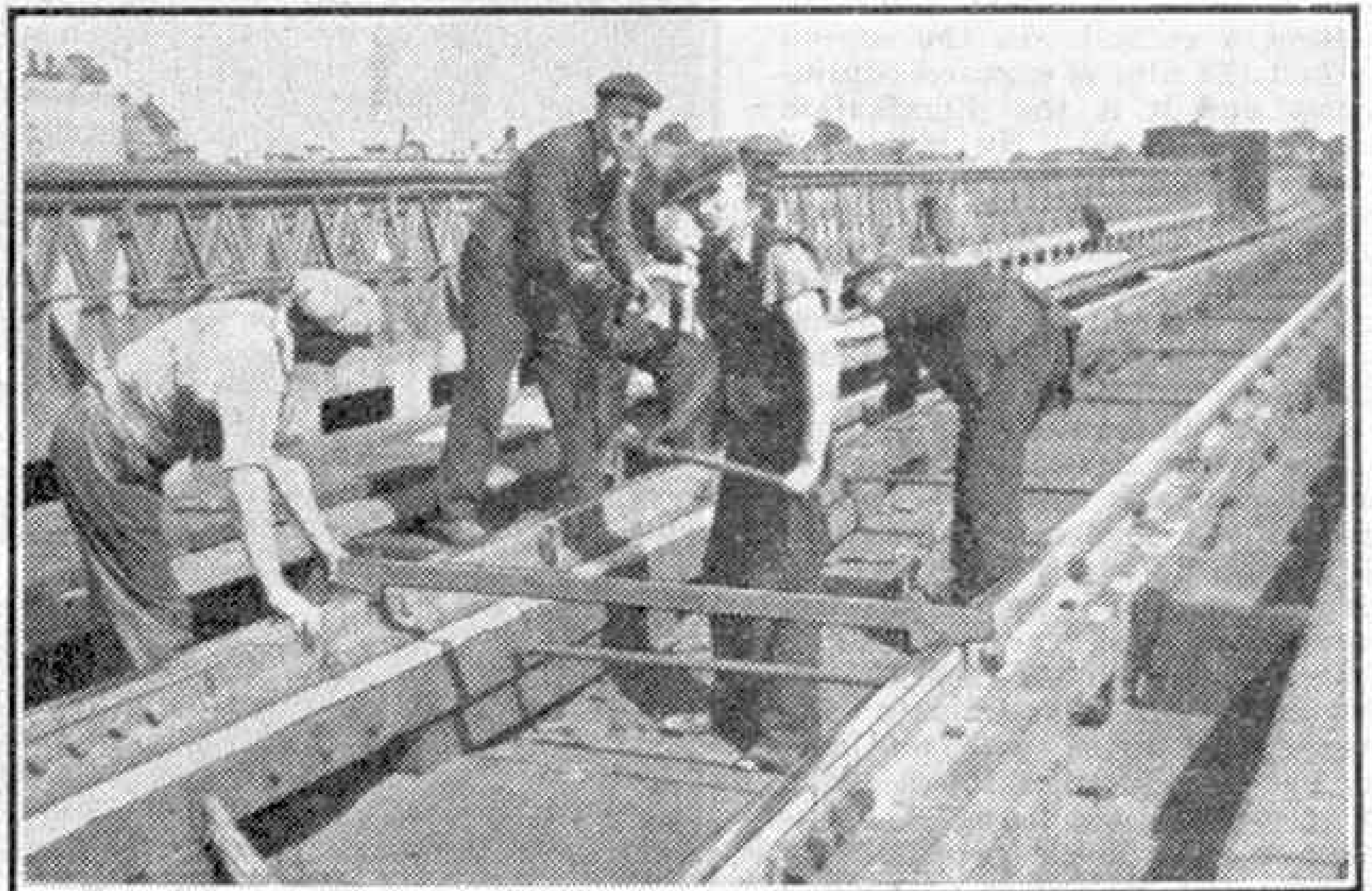
A permanent way gang at work on the track over a bridge. The photograph, by W. Philip Conolly, shows the special form of track construction described in this article.
