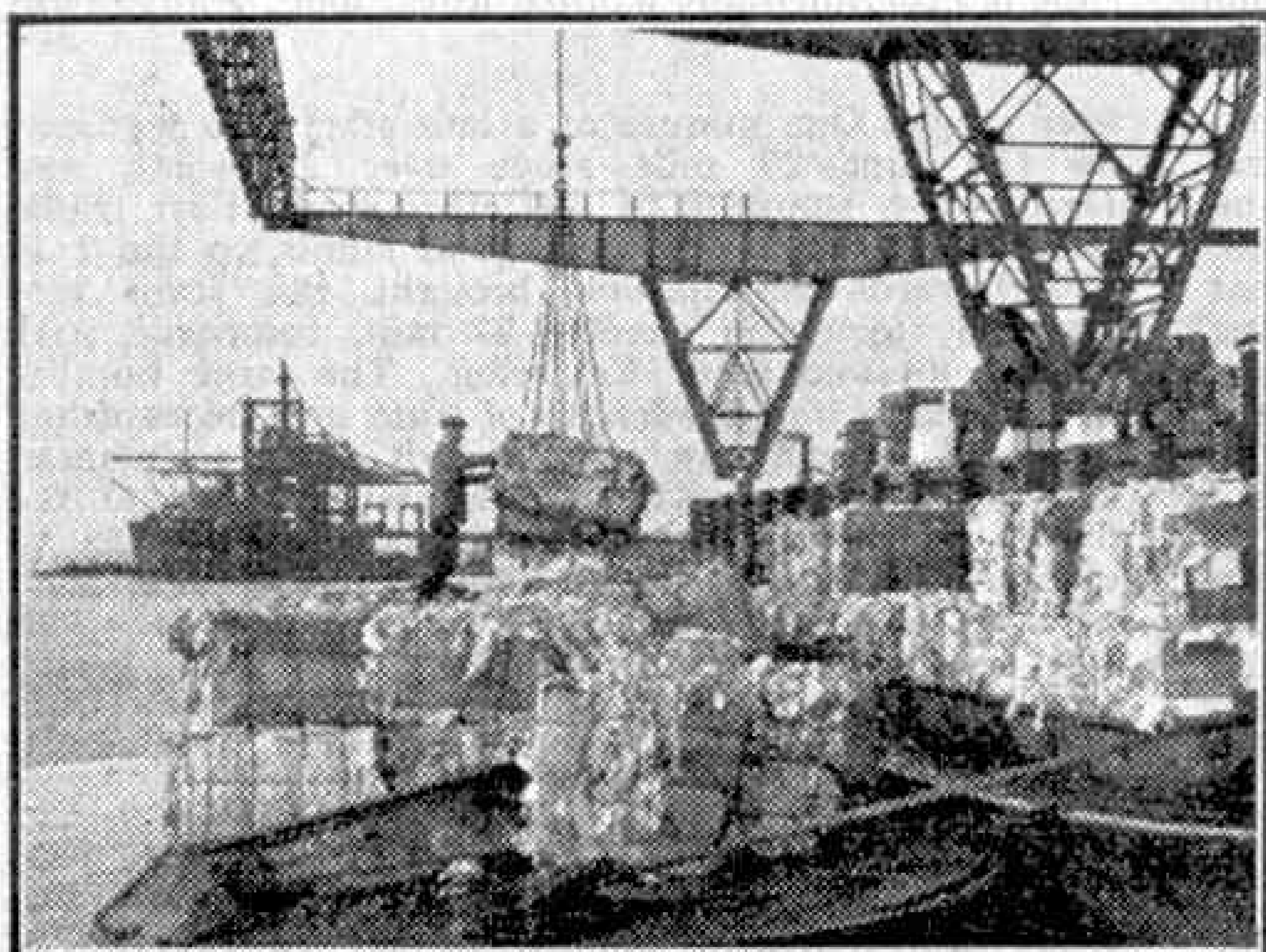
One of the electrically-driven cranes which unload raw material at Thames Board Mills. Illustrations by courtesy of Thames Board Mills Ltd.
