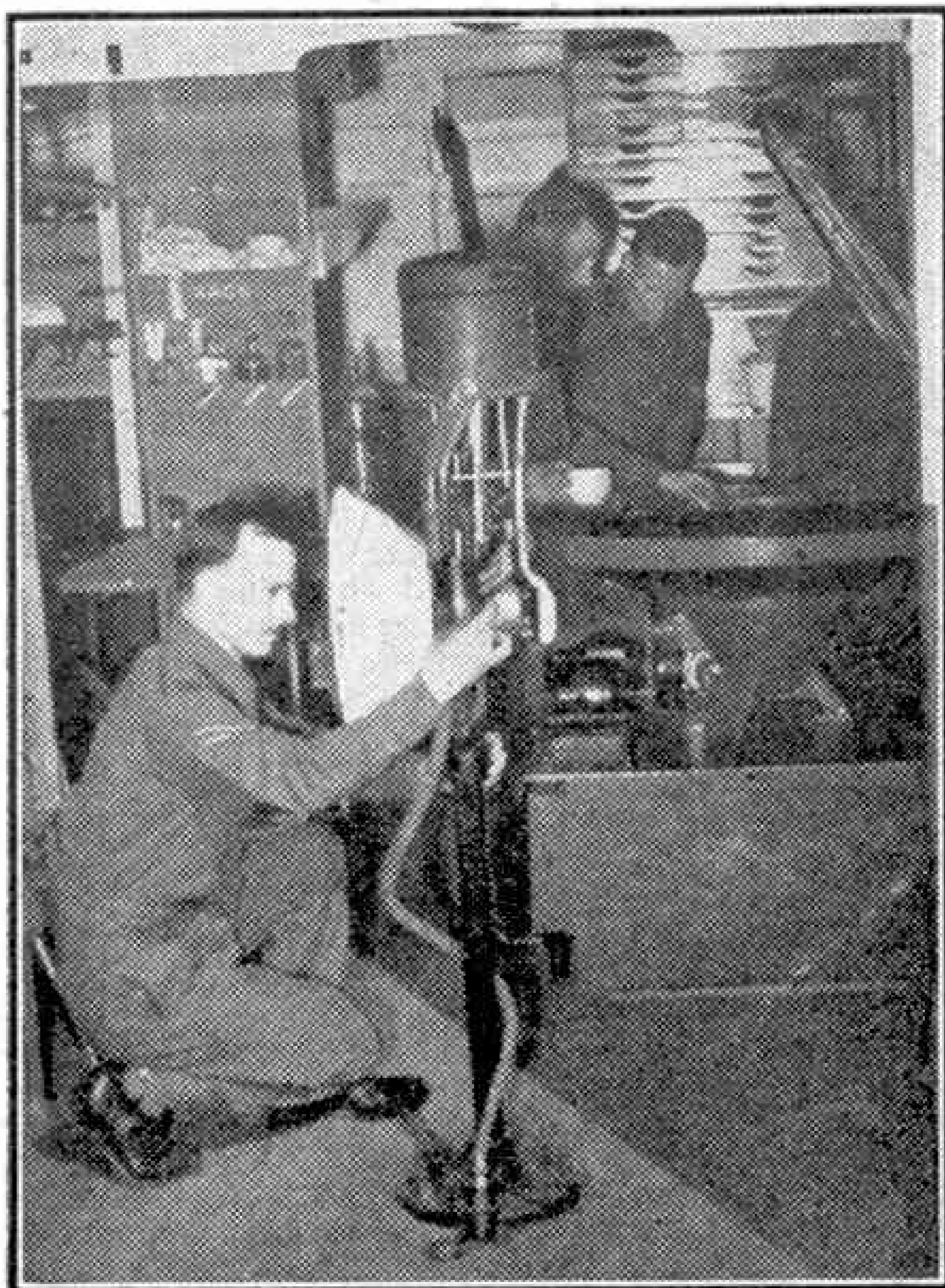
Inside the lorry in which maps are made from aerial reconnaissance photographs. The lamps are being adjusted for making an exposure in preparing the printing plate.
